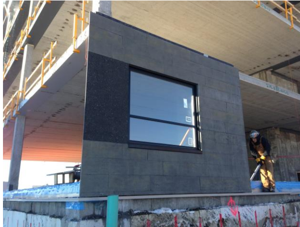
Figure 2. Installation of precast concrete walls with pre-installed windows at the factory
