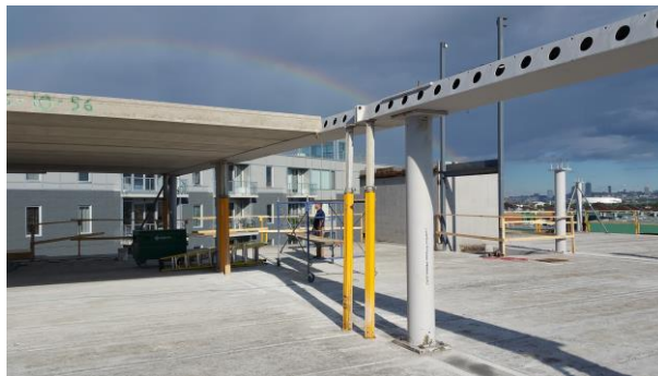
Figure 1. On-site assembly of the new slim-floor system
