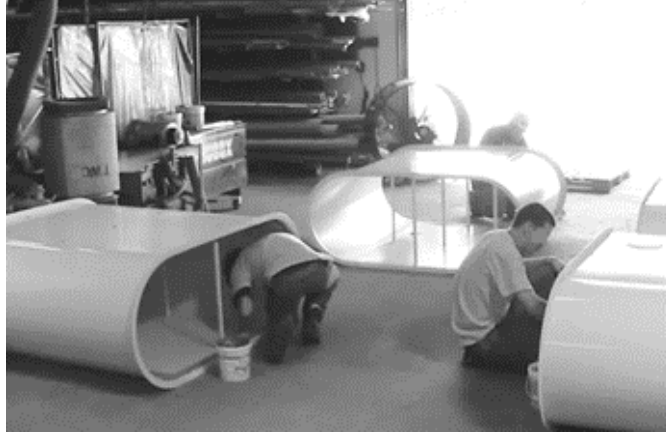
Figure 2: Sheet metal ducts sealing task performed by three workers
