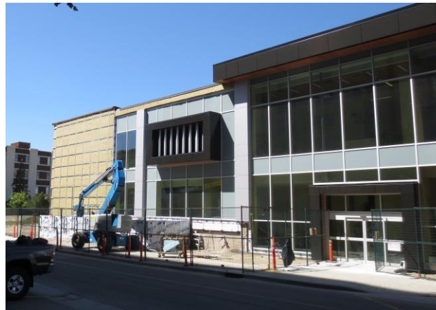
Figure 4. Building envelope retrofit of the John Ware building on SAIT campus
