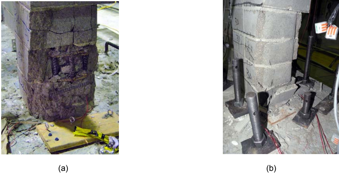
Figure 4. Wall failure: (a) bar buckling and grout crushing in wall 4 at 13\Delta_y , (b) vertical cracks in the boundary element in wall 5 at 11\Delta_y .
