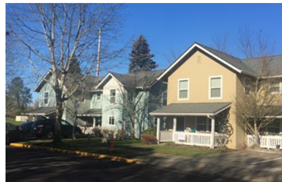
Figure 2: A view of typical housing in the Camas Commons project
