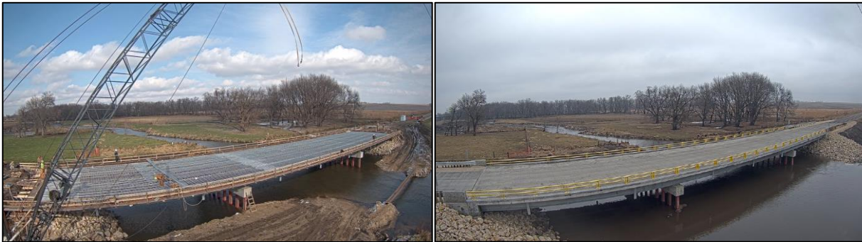
Figure 3: Buffalo Creek Bridge in Independence, Iowa
