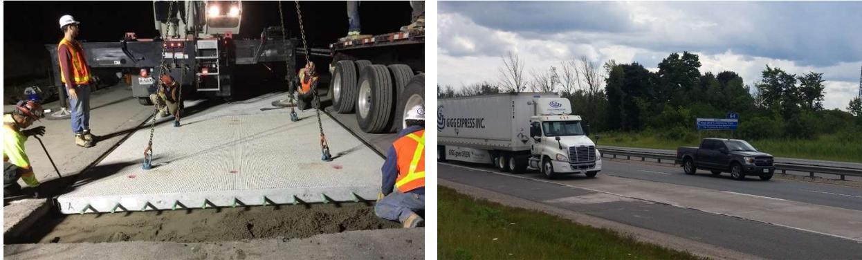
Figure 1: Precast concrete inlay panels installation in third lane on Highway 400 during construction (left) and in service (right)
