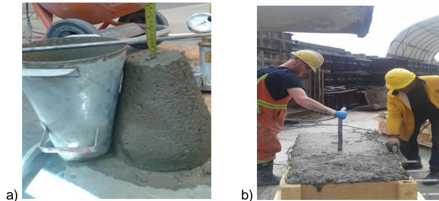
Fig 1 Concrete pouring a) slump testing and b) internal concrete vibration
