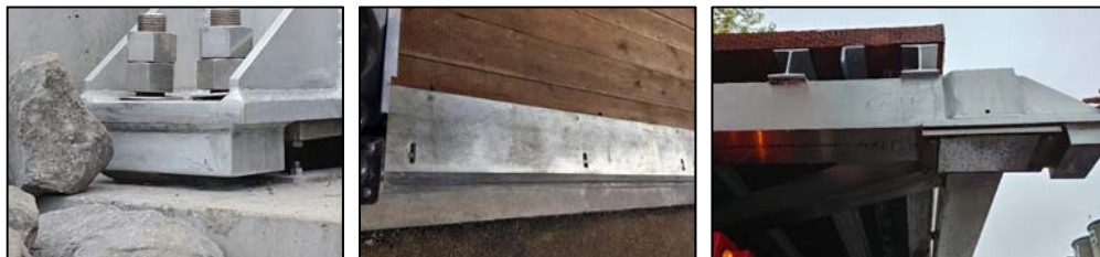
Figure 2: From left to right: anchorage rods, expansion joint and sliding bearing devices
