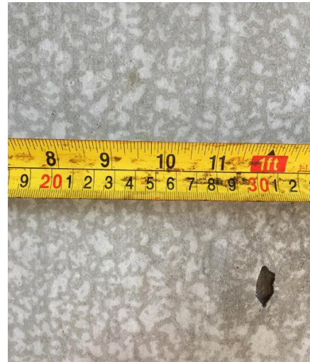
Figure 2: Box culvert surface Meatbird Creek, 2018, 96-hour cure by water immersion
