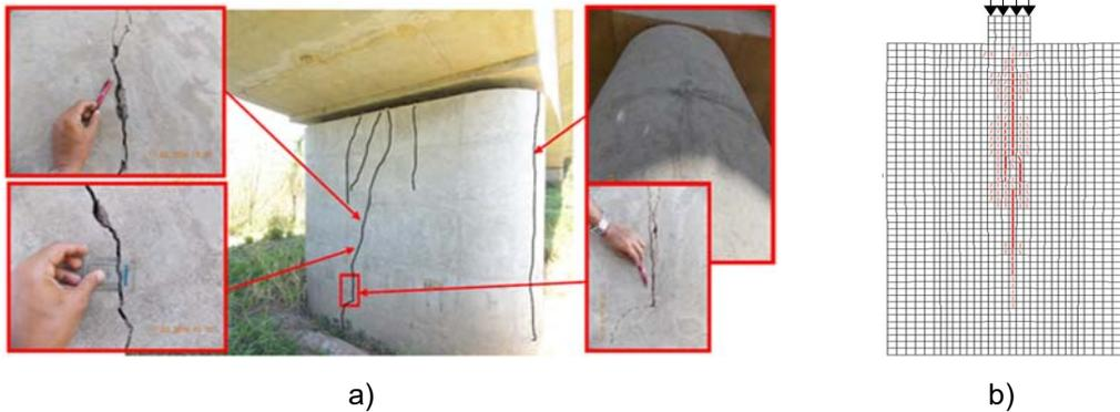
Figure 4. Cracking patterns: a) Real structure (eBridge, 2016), b) Model structure
