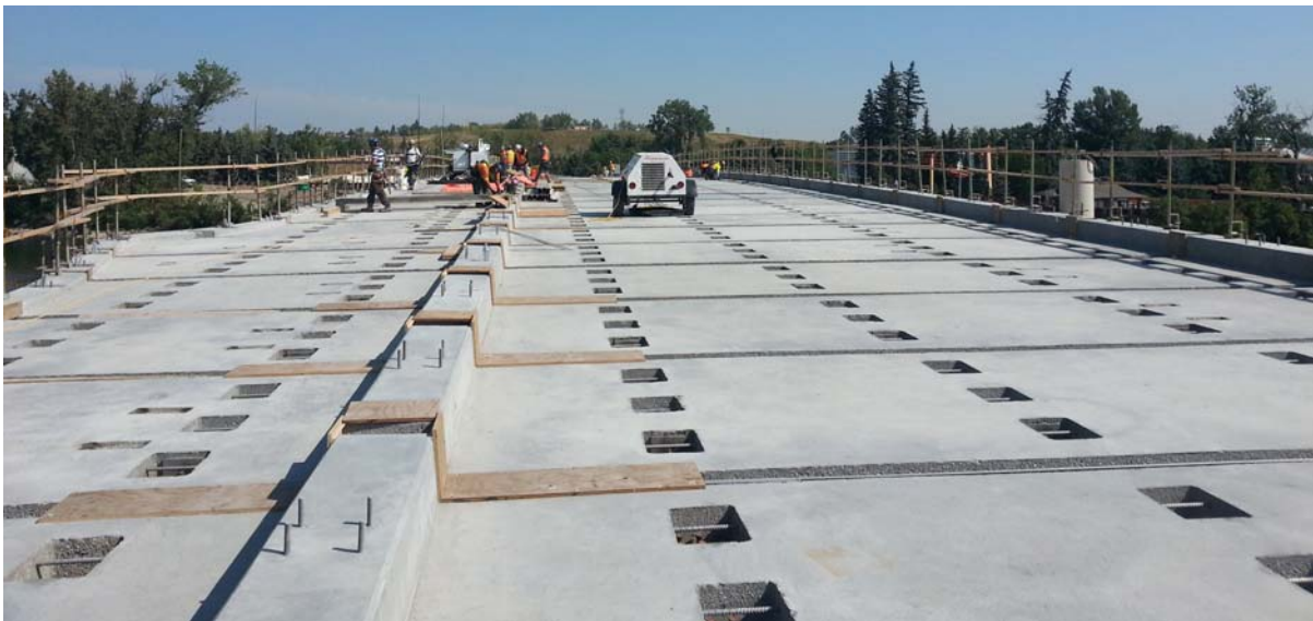
Figure 8: Full-depth, full-width, precast deck panels installed on the bridge
