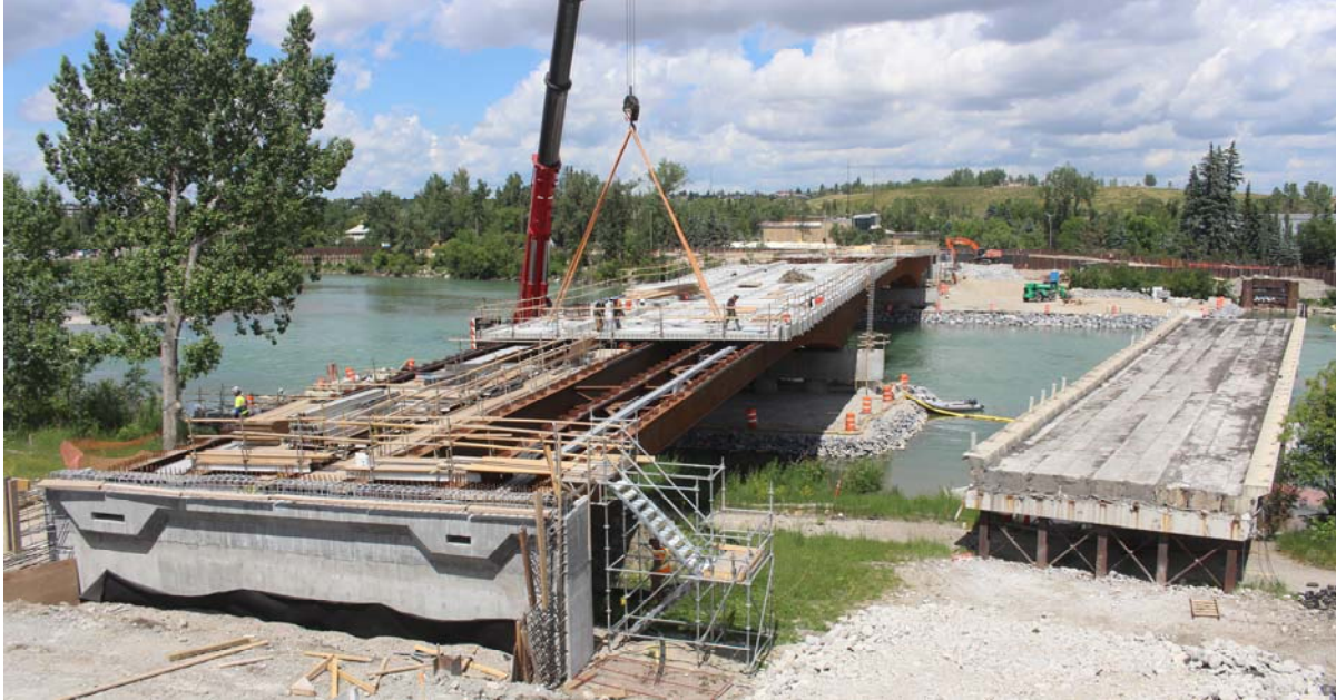
Figure 7: Panel erection
