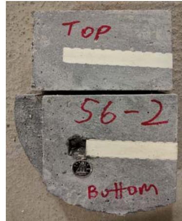
Figure 15: View of bar slippage failure in slab S6 due to shearing of the bar ribs and bar slip
