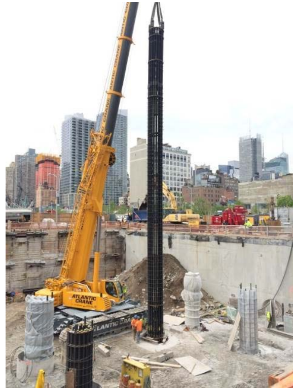
Fig. 10: b) 55 Hudson Yards_ Caisson splicing
