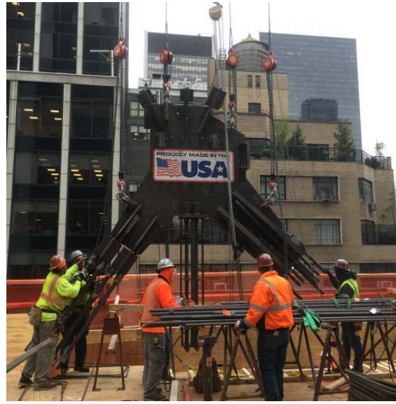
Fig. 12: b) Node erection and installation
