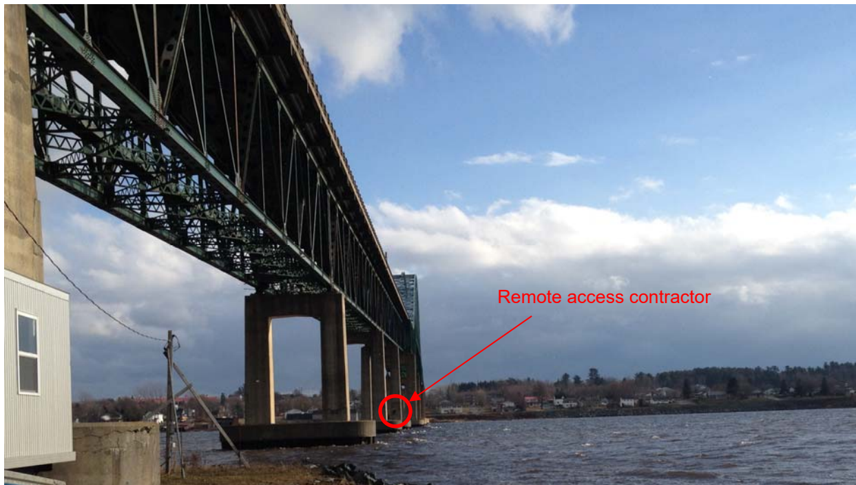
Figure 2: Remote Access Contractor Drilling Core from Concrete River Pier
