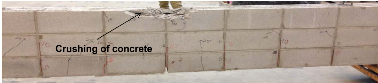
Figure 7: Failure of beam specimen 30-S-N
