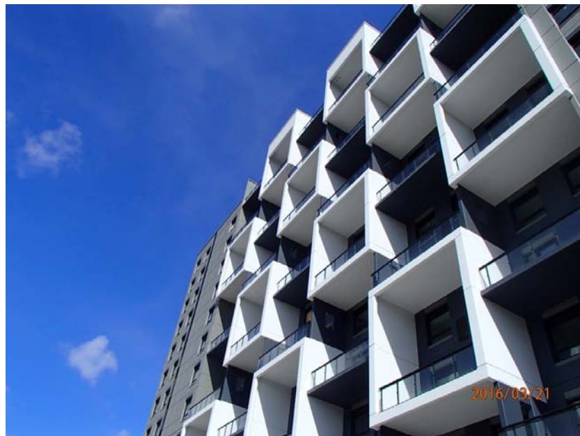
Figure 3: Completed Building Facade
