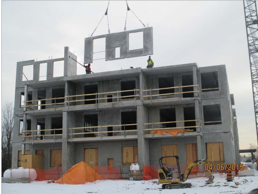
Figure 1: Erection of a Typical Wall Panel (Winter Construction)
