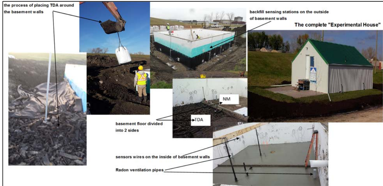
Figure 2: the Experimental House during and after construction
