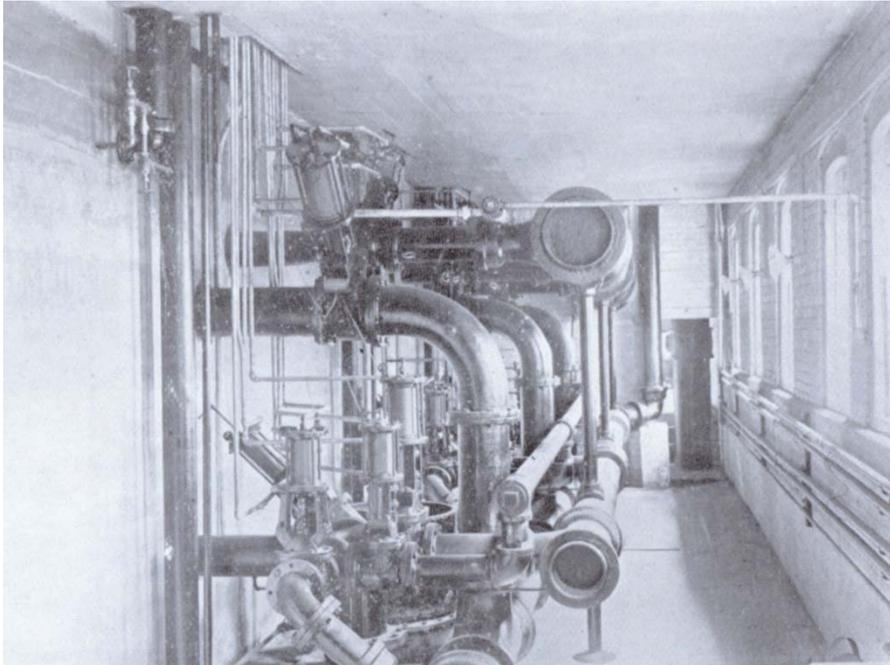
Figure 4: Piping to and from the three rapid sand filters at the Fredericton Pumping Station and Water Treatment Plant (c. 1906).
