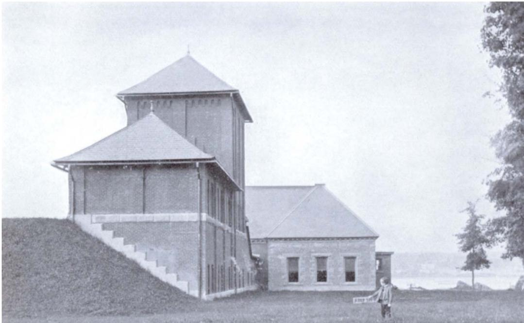
Figure 3: Fredericton Pumping Station and Water Treatment Facility (c. 1906). The tall tower houses the constant head tank for the rapid sand filters in the lower portion of the building. [Source: Provincial Archives of New Brunswick Image: P657-25]
