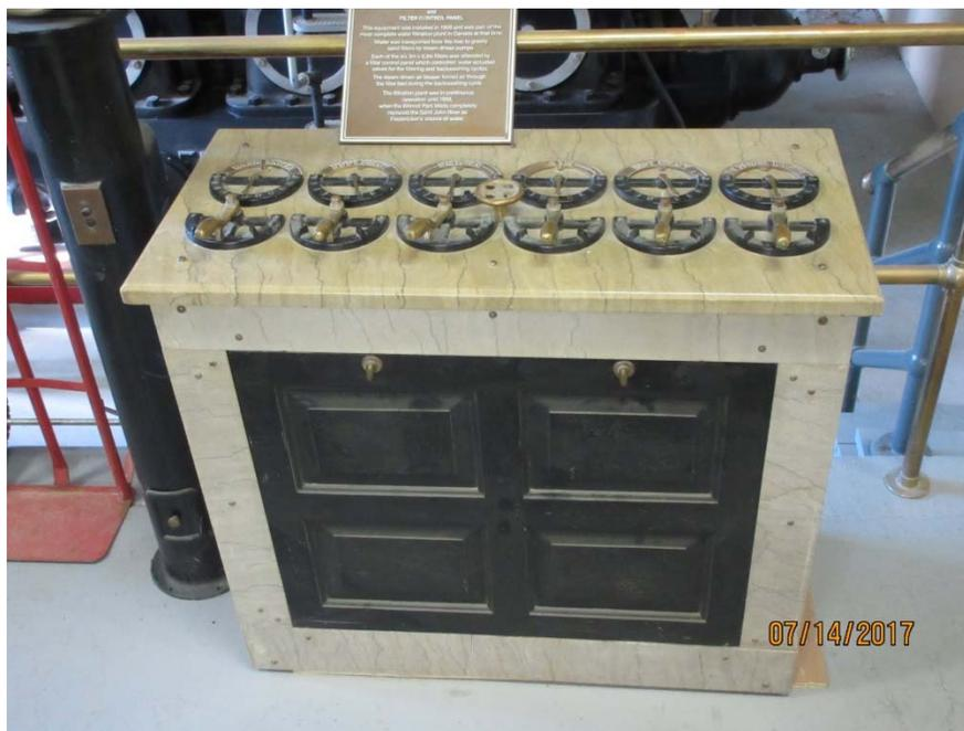
Figure 5. An original control panel for the rapid sand filter for the 1906 plant.
