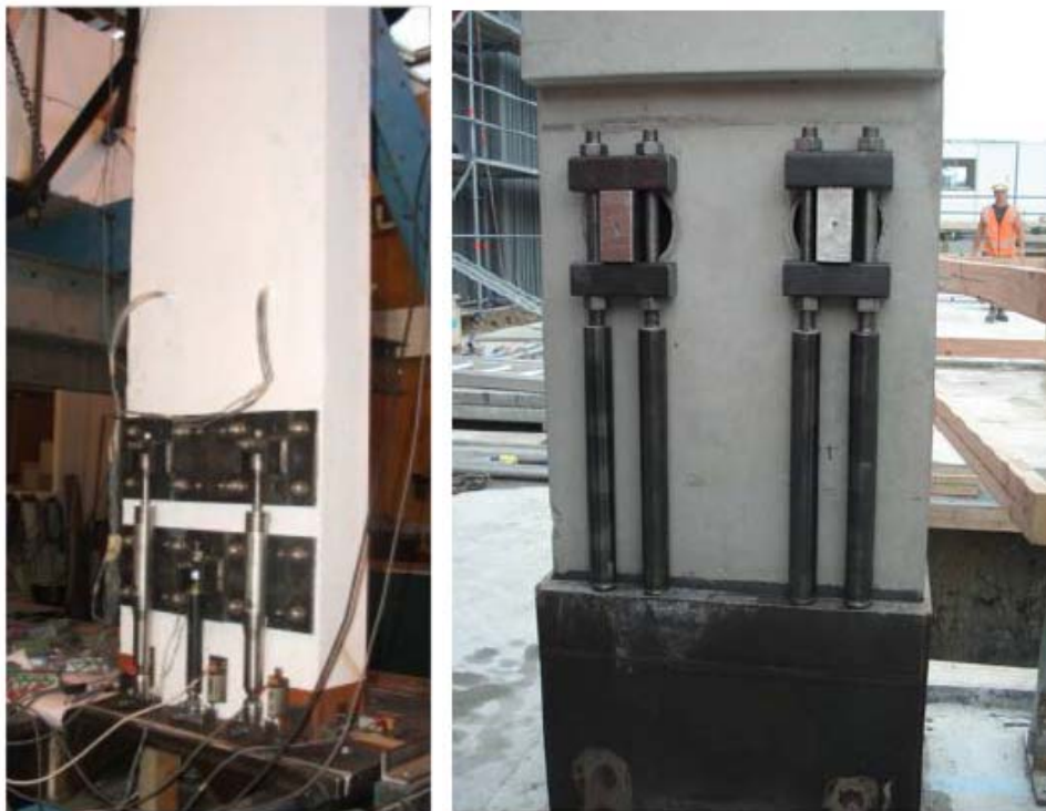
Figure 4: Example applications of Hybrid concept in practical concrete structures (Pampanin et al. 2012a)
