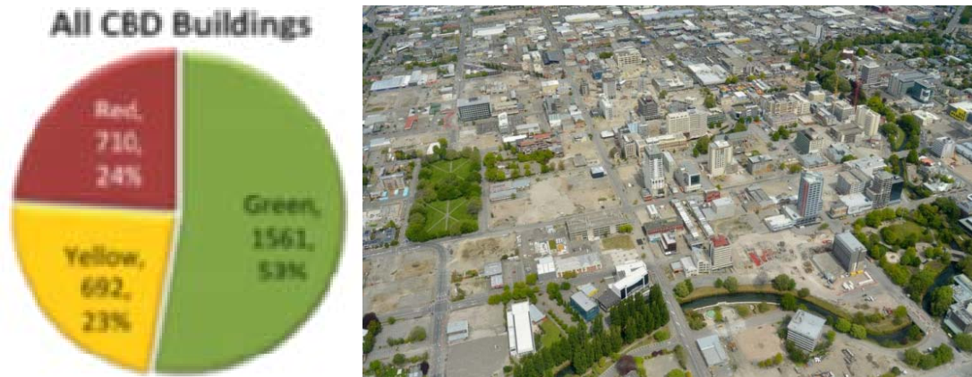
Figure 1: Distribution of building designations in Christchurch CBD after the earthquakes in 2010-2011 (Kam et al 2011, left) and aerial view of the CBD with empty lots after demotion (Pampanin 2012b)
