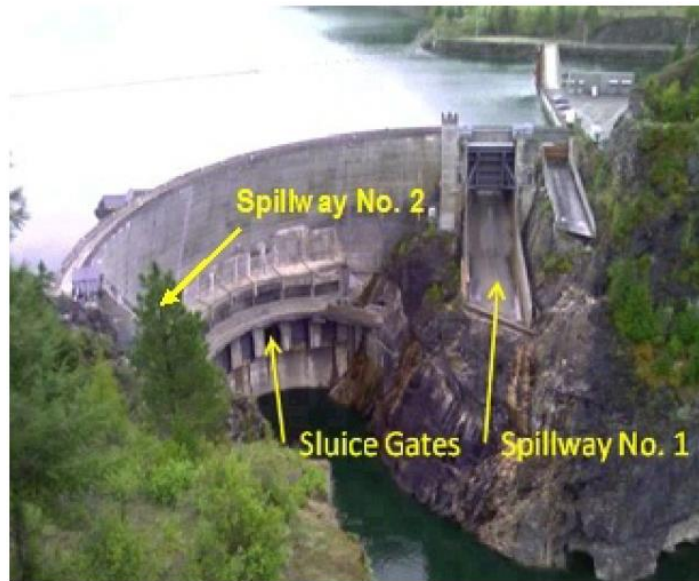
Figure 2 Downstream View of Boundary Dam Looking Upstream
