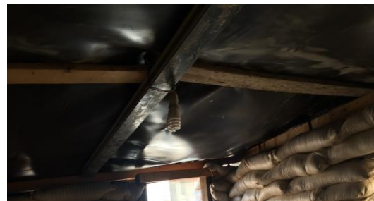
Figure 2: High-density polyethylene sheets on wooden frame roof system
