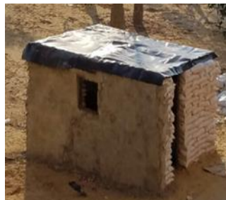
a) External view of he constructed room
