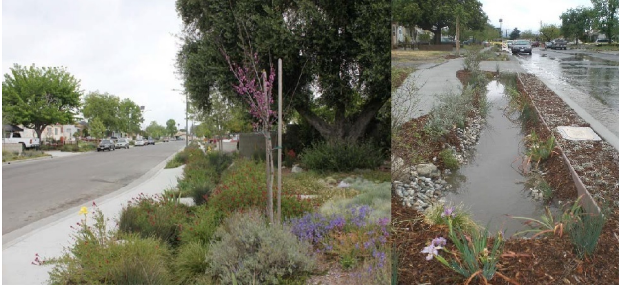
Figure 1: Typical Roadside LID BMP Installations (Amec Foster Wheeler)
