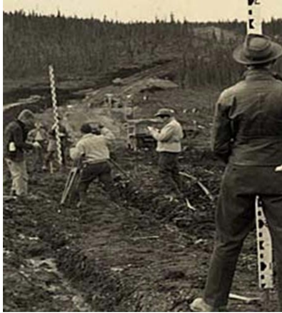
Figure 4: Surveying of Alaska Highway during reconstruction work
