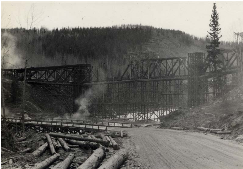
Figure 3: Kiskatinaw Bridge near Dawson Creek was built in 1942 to replace timber trestle (in foreground)
