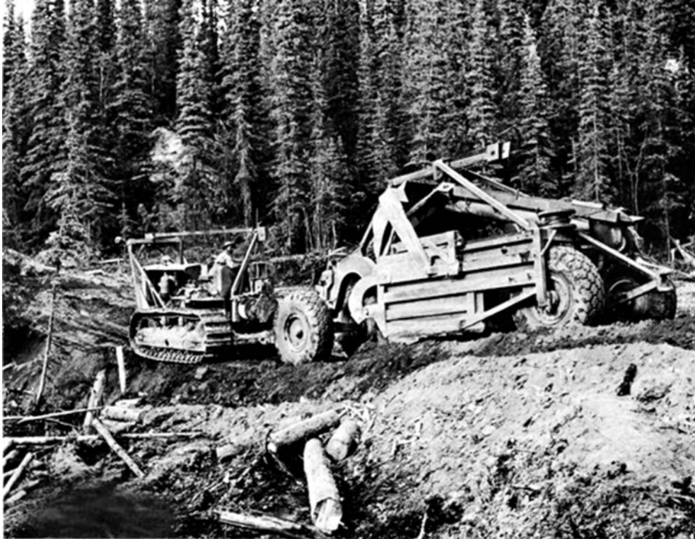
Figure 2: Operating a scraper during the original construction of the Alaska Highway
