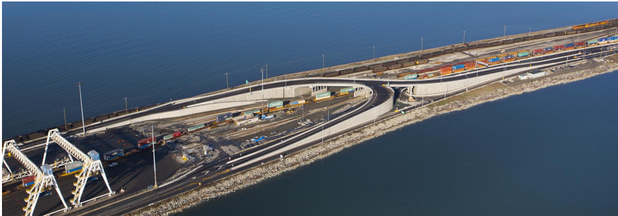
Figure 1: Deltaport Causeway Overpass, Vancouver, B.C.
