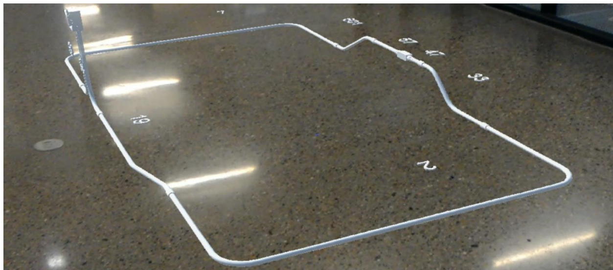
Figure 3: Electrical conduit as viewed from the HoloLens, placed on the ground
