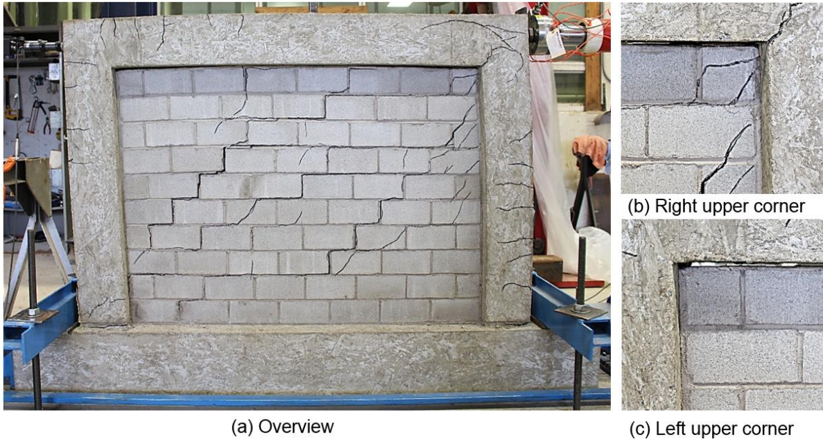
Figure 7 Failure pattern of specimen IFTG12
