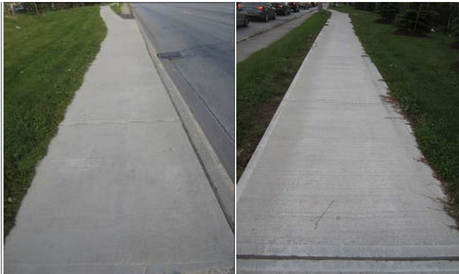
Figure 12: Site Condition – Control Mix (1 Year)
