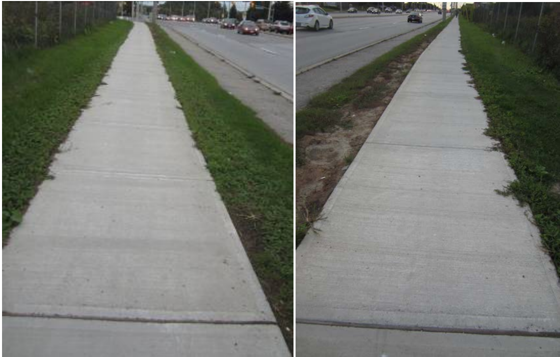
Figure 13: Site Condition – 20% Granular Mix (1 Year)
