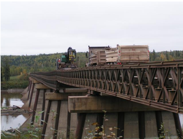
Figure 2: Vehicle Convoy Crossing Bridge
