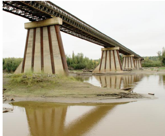
Figure 3: View of Bridge from River Level
