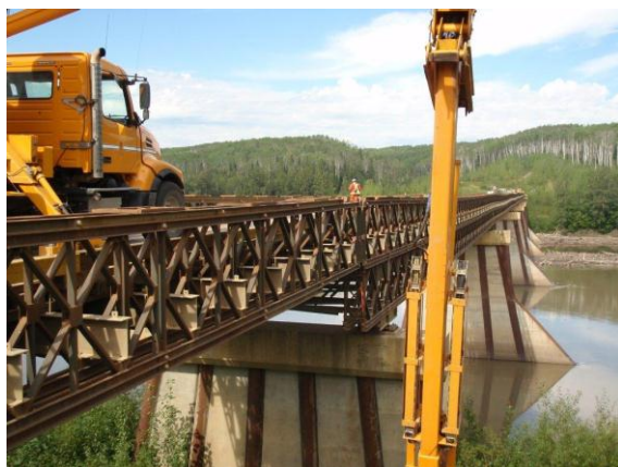
Figure 4: Bridge Inspection Using Snoopers Truck
