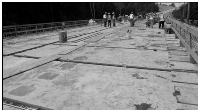
Figure 5: GFRP in precast panels and barrier walls (Young et al. 2012)
