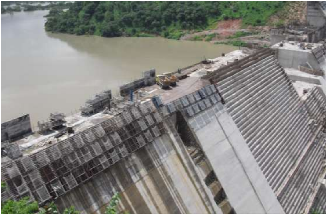
Figure 4: RCC dam construction in Ghana (Schiffler, 2014).
