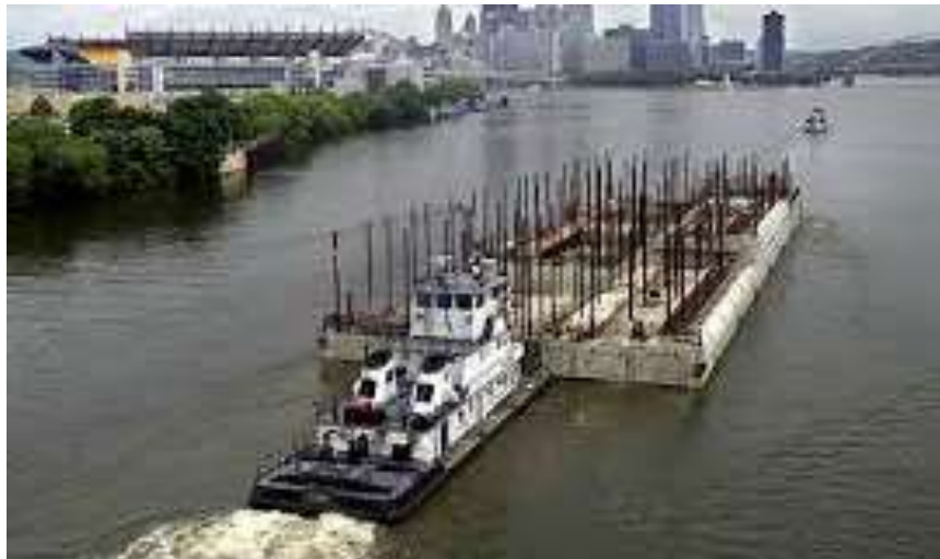
Figure 6: Floating the dam segments (Bittner-Shen Inc., 2013).
