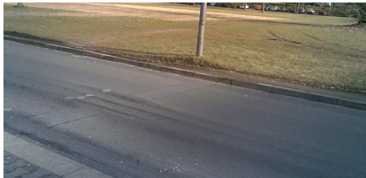
Figure 2: Rut formation along the wheel track
