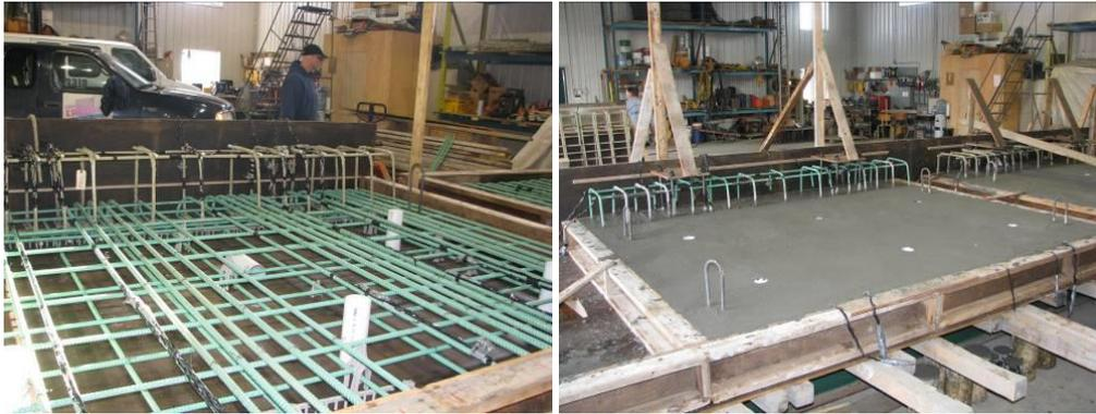
Figure 2: Fabrication of the barrier prototypes
