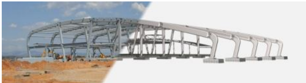
Figure 3: Example of LOD 400 for structure, real picture of the works and the BIM model compared
