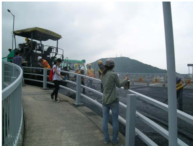
Figure 3: Measurements of VOCs during the paving stage
