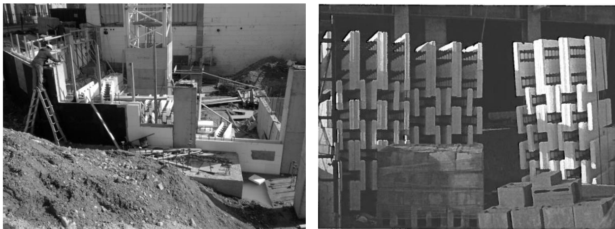
Figure 3: Polystyrene foam formwork block (Waterloo, 2011)
